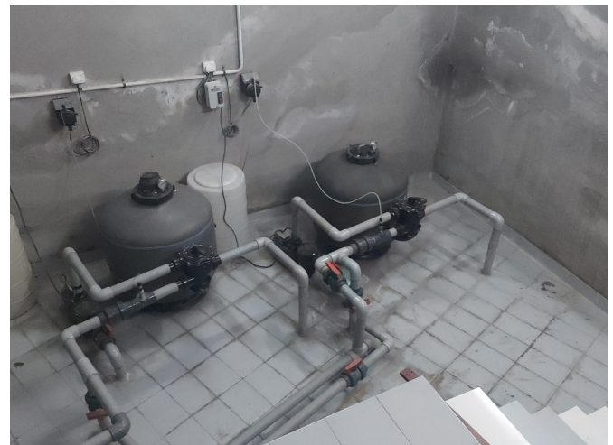
The 44kW Electroheat Plus Heat Pumps (left), Micron Side Mount SM750 Filters and Supatuf MK2 Pumps (right) installed at Centra Greens
