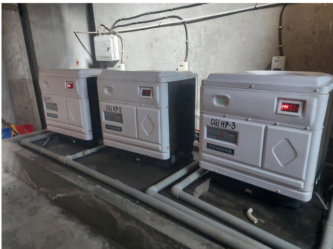
The 44kW Electroheat Plus Heat Pumps (left), Micron Side Mount SM750 Filters and Supatuf MK2 Pumps (right) installed at Centra Greens
